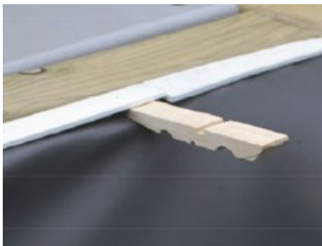
Figure 31 – Blocking the liner in position using half clothes pegs
