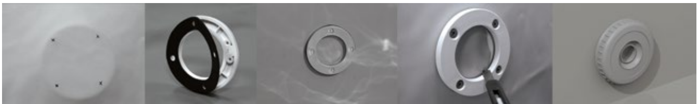
Figure 34 – Installing the return fitting flange
