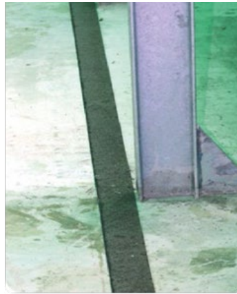
Figure 8 – Laying the bituminous strips
