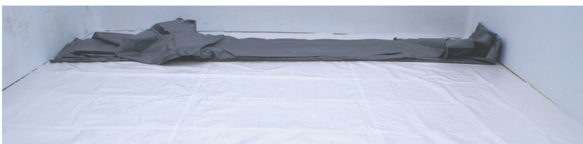
Figure 32 – Unfolding the liner
