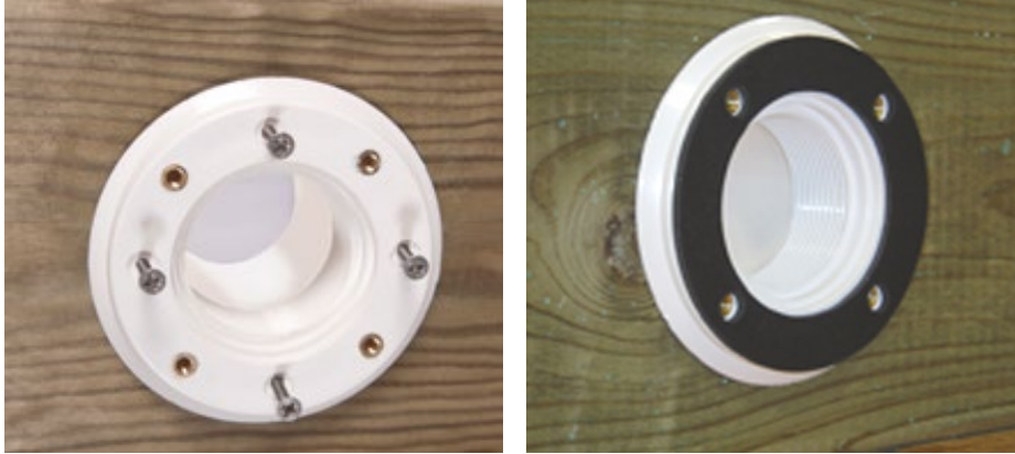
Figure 23 – Mounting the return fitting body and gasket
